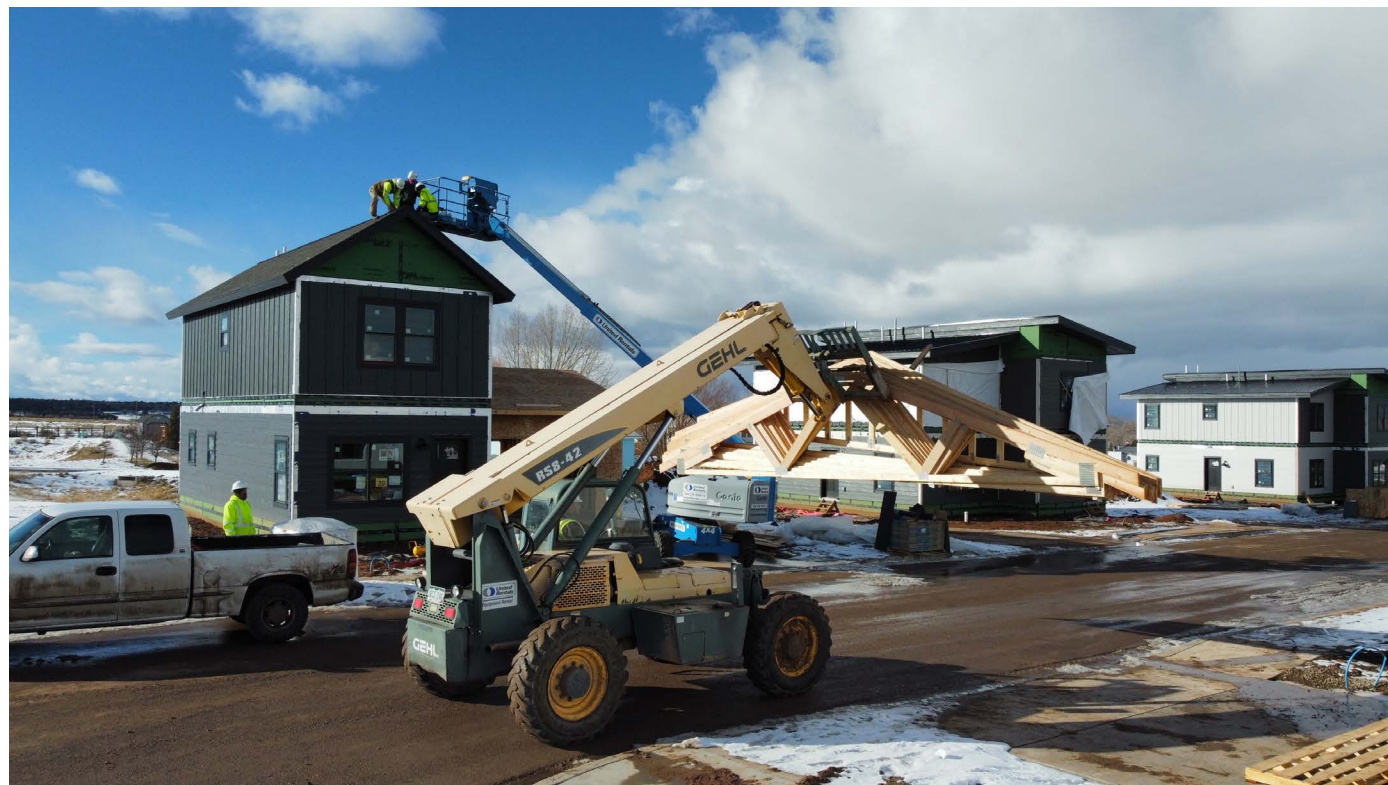
Step 7: on site finish including garages, porches, and solar panels!
