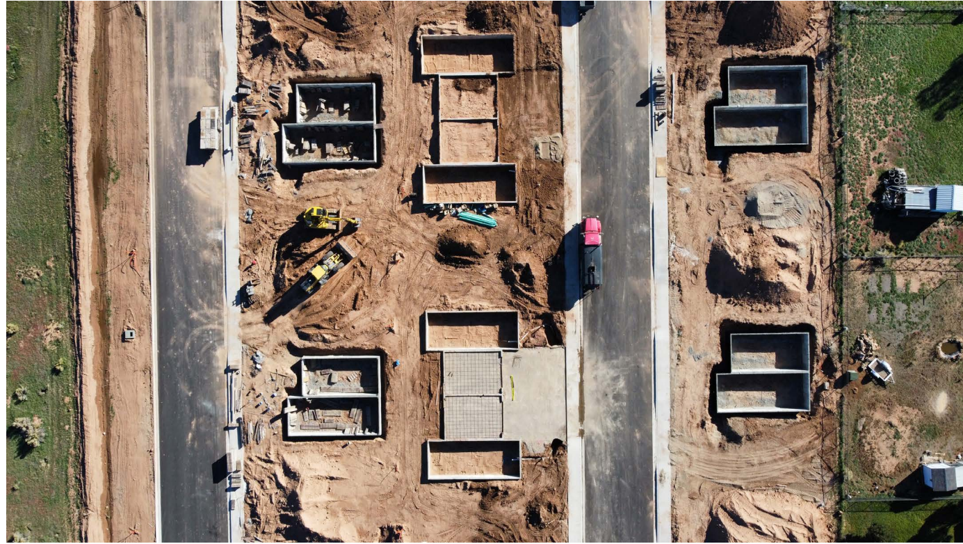
Step 1: site work - including foundations & infrastructure
