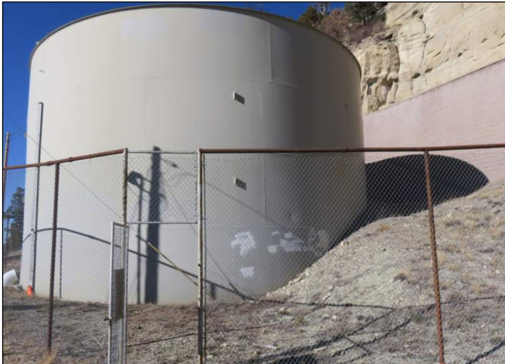
Figure 4-2. Existing Storage Tank
